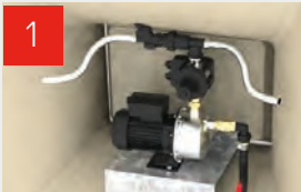
1 Pump pre-installed with rain/mains changeover
